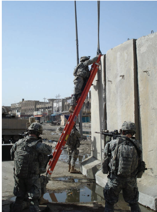
Figure 5.4 Unhooking a T-Wall Section
