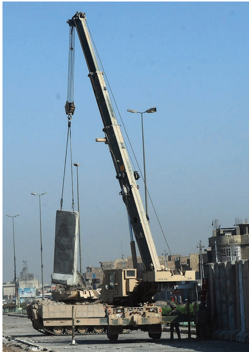
Figure 5.3 Emplacing a T-Wall Section
