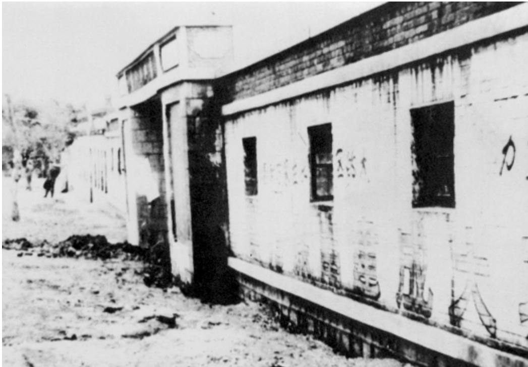
Figure 65. Uneven settlement of office building, Fankenchuang Commune, Luan-nan hsien.
