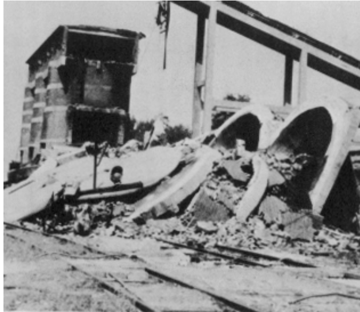
Figure 55. Collapsed brick cylindrical storage bin at the Fankechuang mine.
