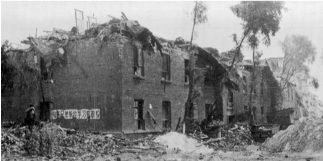
Figure 43. Collapsed top story of the three-story Kailuan coal mine dormitory, Tangshan.
