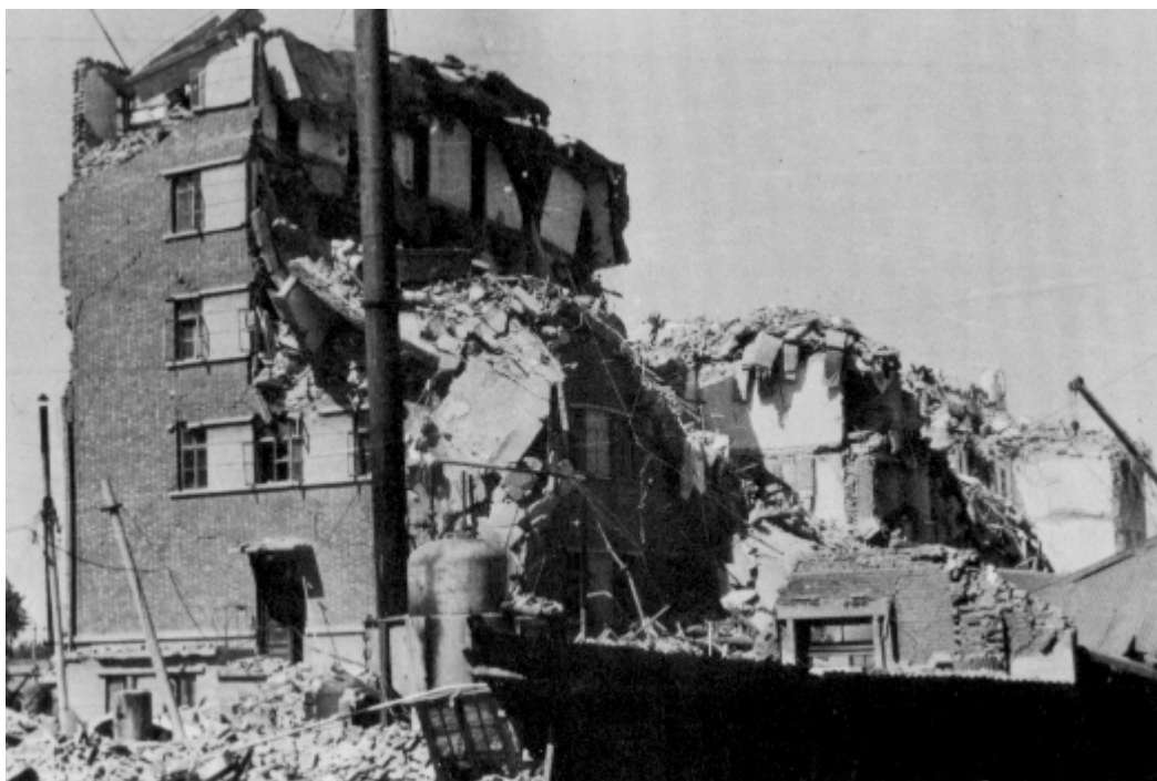
Figure 46. Collapse of Kailuan coal mine reception building, Tangshan.
