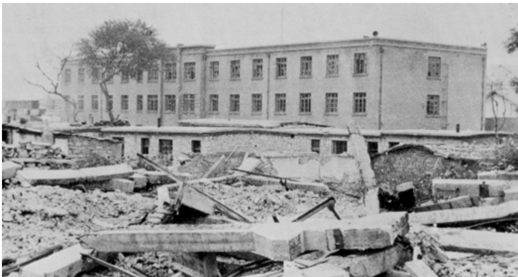
Figure 70. Tangshan light-machine plant official building. This structure, which was located in district 13 of Figure 39, was only slightly damaged. The remains of a collapsed building can be seen in the foreground.
