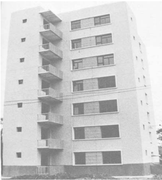
Figure 10. Nearly completed seven-story apartment building in Chengdu. The building has brick bearing walls and precast concrete floor slabs.
