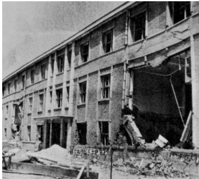
Figure 66. Damaged building at Kailuan coal mine general hospital in Tangshan.
