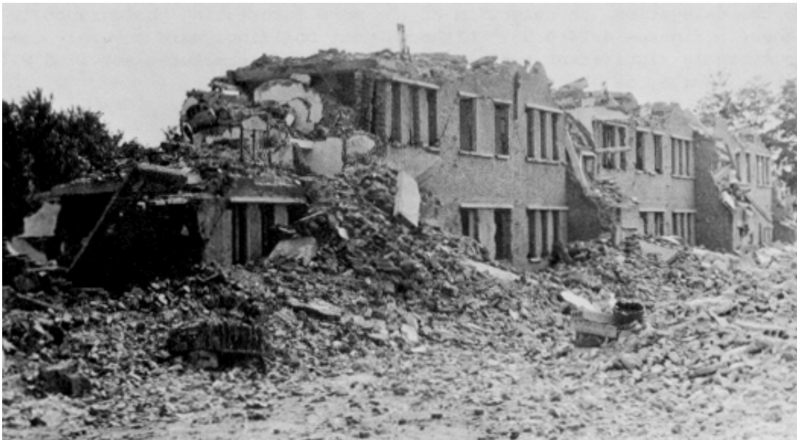
Figure 44. Collapsed four-story Tangshan Mine-Metal Institute residence building.
