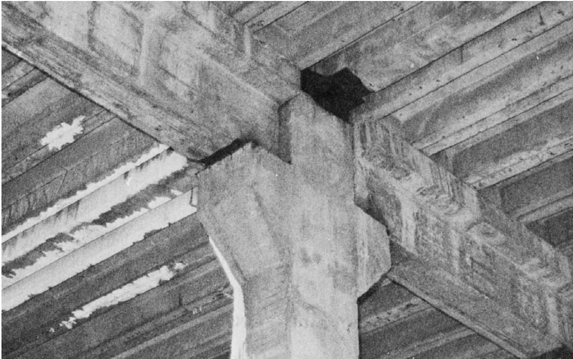
Figure 18. High one-story portion of Chengdu industrial building was of precast concrete construction. The roof slab was composed of precast concrete channel sections.
