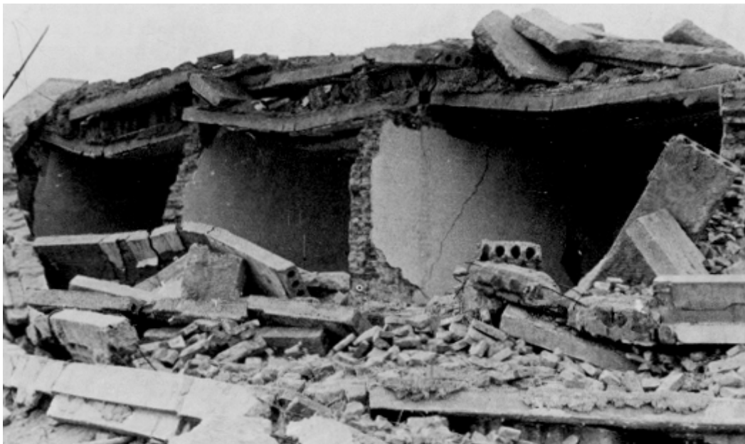
Figure 53. Collapsed building showing the type of construction: precast concrete floor slabs made of four-hole beams, simply supported on bearing walls.
