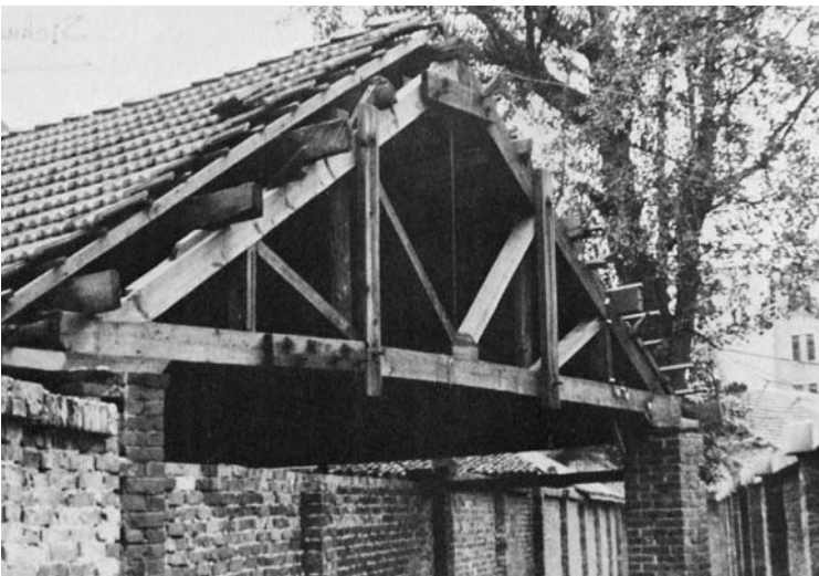
Figure 11. Timber truss on a small building in Chengdu near the apartment building of Figure 10. Note the unreinforced brick columns, which appeared to be used extensively in China.
