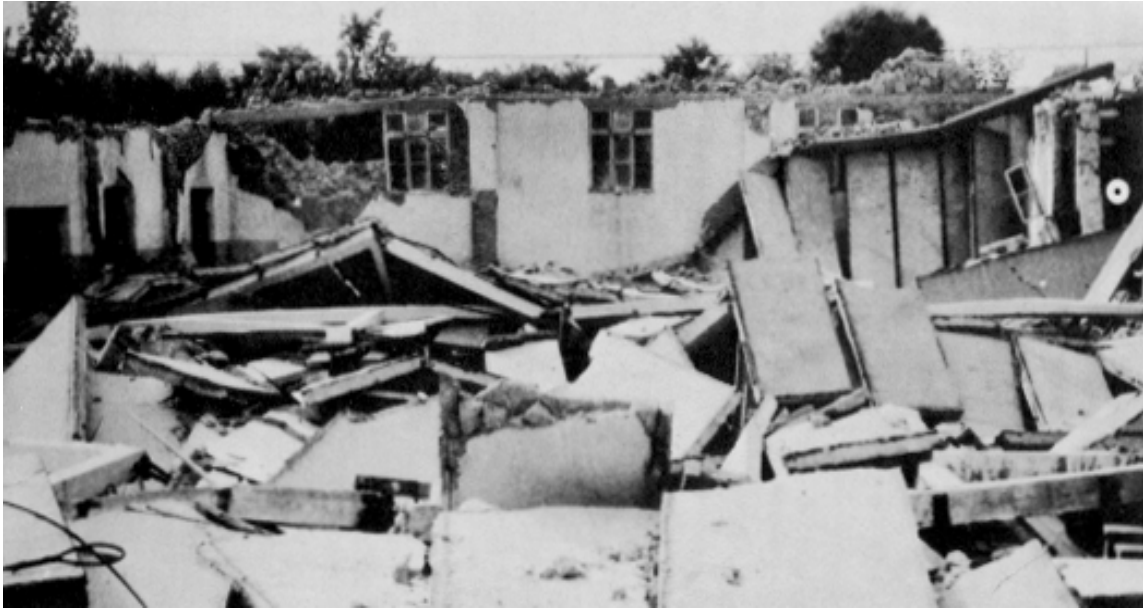
Figure 51. Collapsed workers' cafeteria building of the Chinkechuang coal mine.
