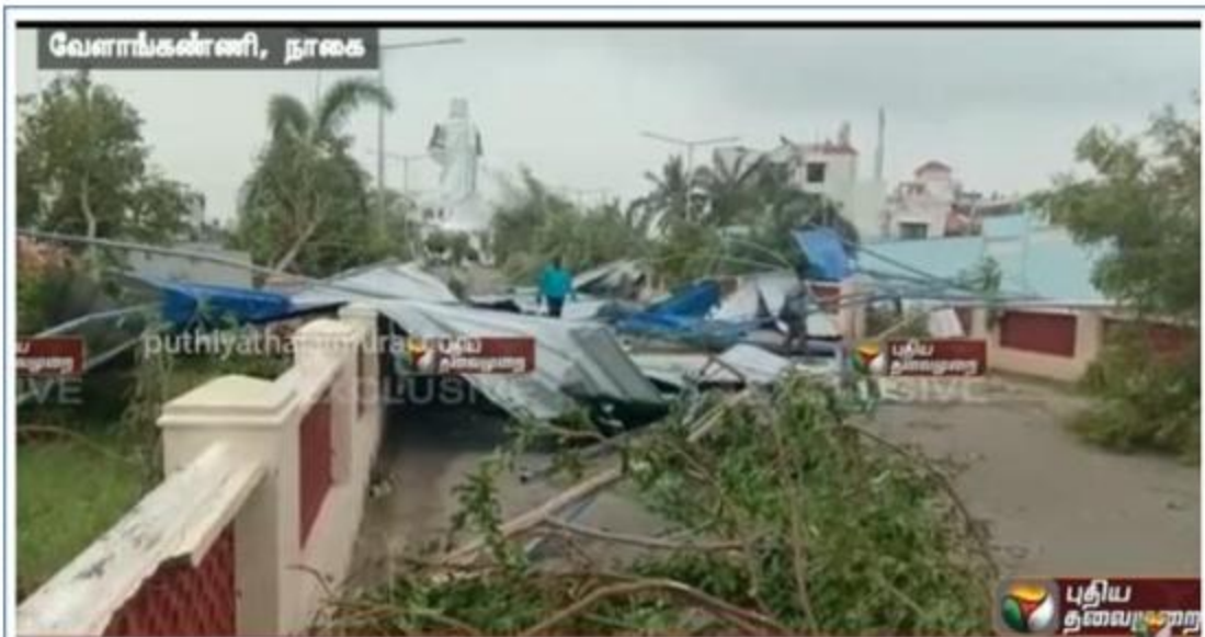
Damaged structures and fallen trees in Velankanni, Nagapattinam district (Source: puthiyathalaimurai.com)
